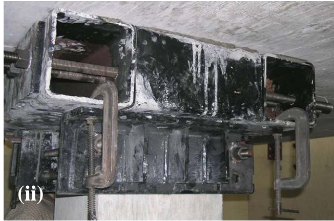
Figure 4.10 Installation of the angles
