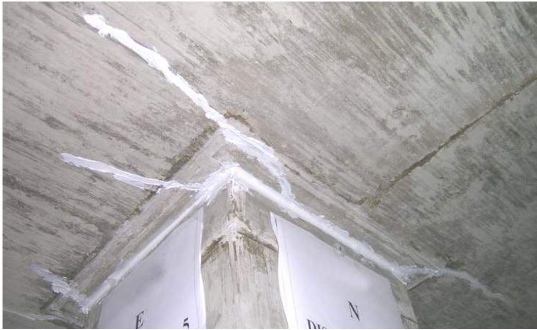
Figure 4.38 Cracks were sealed with silicone
