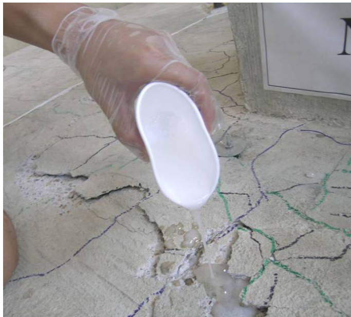
Figure 4.13 Pouring epoxy into cracks
