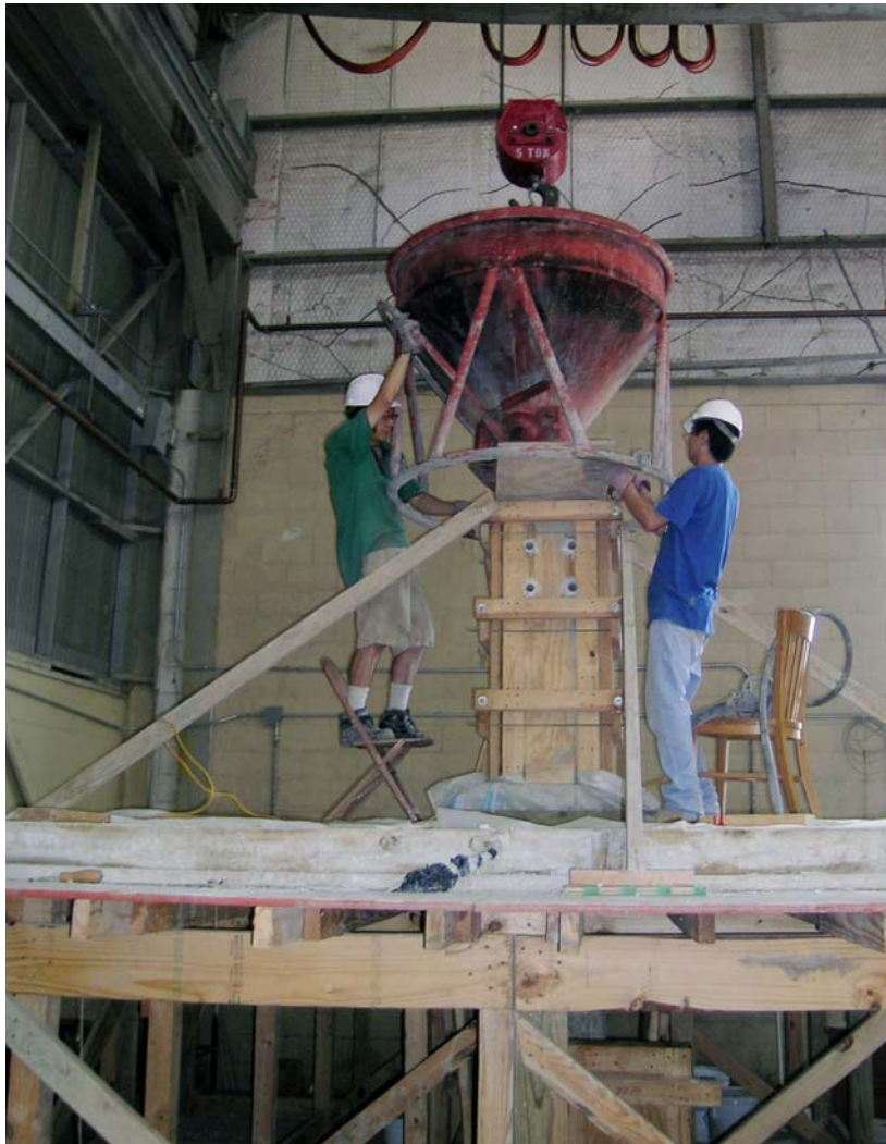
Figure 3.15 Concrete placement: upper column
