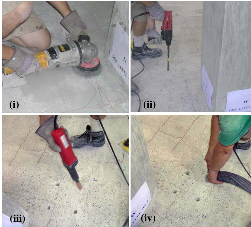
Figure 4.36 Surface preparation before the application of CFRP sheets
