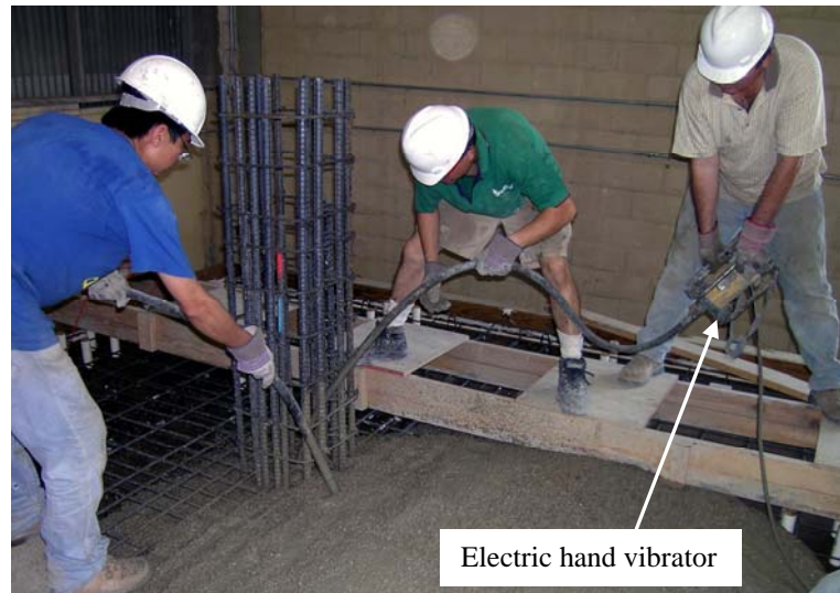
Figure 3.13 Compacting concrete
