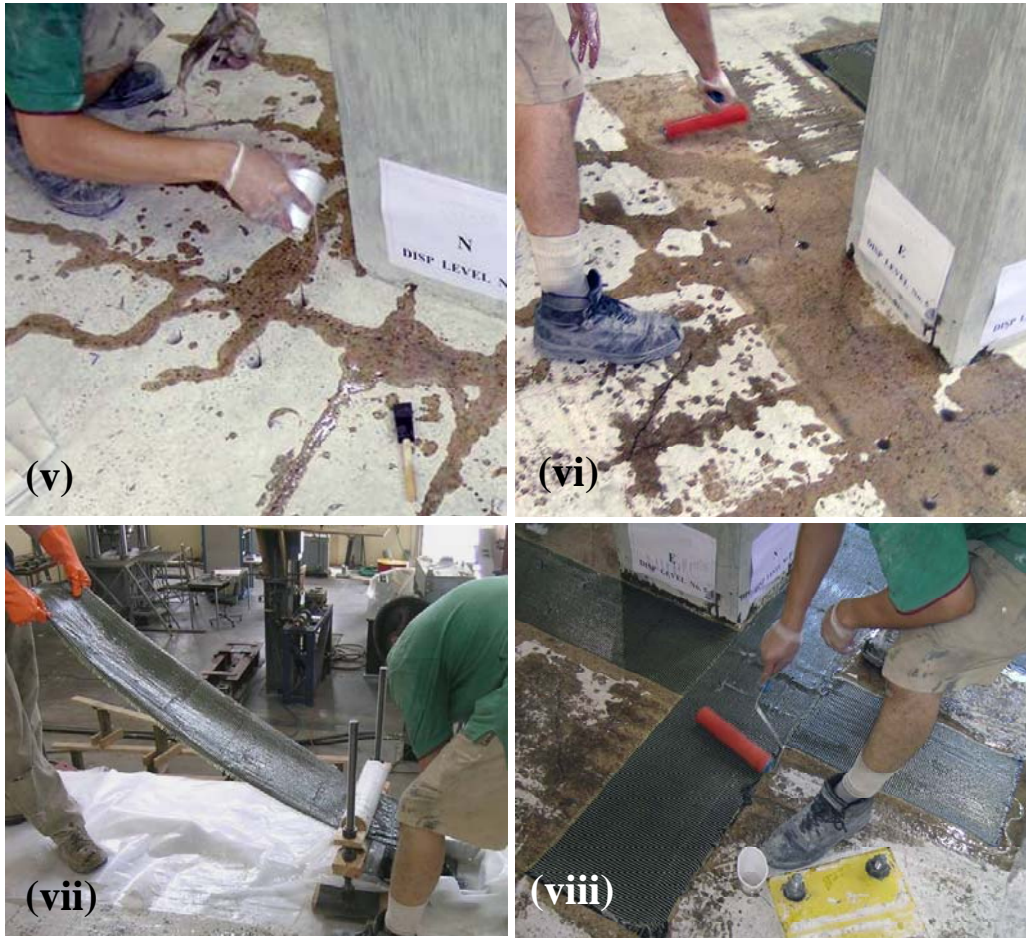
Figure 4.39 Installation of CFRP sheets
