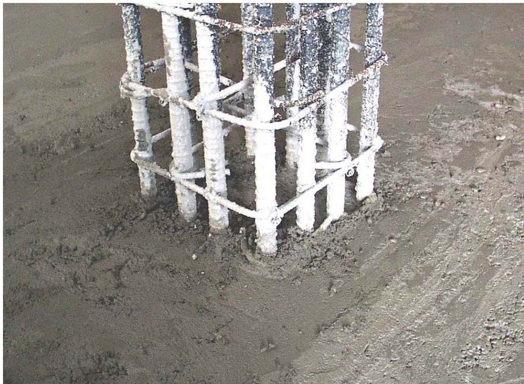
Figure 3.14 Construction joint at slab-column connection
