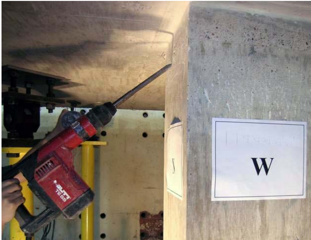
Figure 4.6 Roughening the column surface
