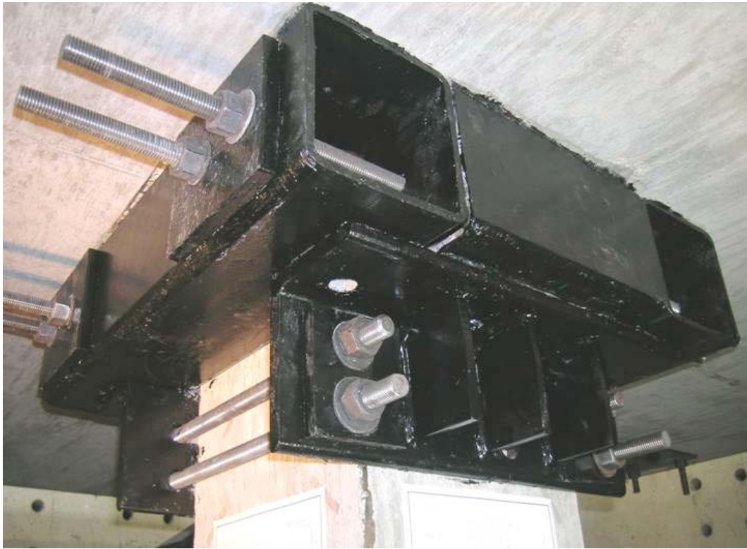
Figure 4.4 Collar after installation
