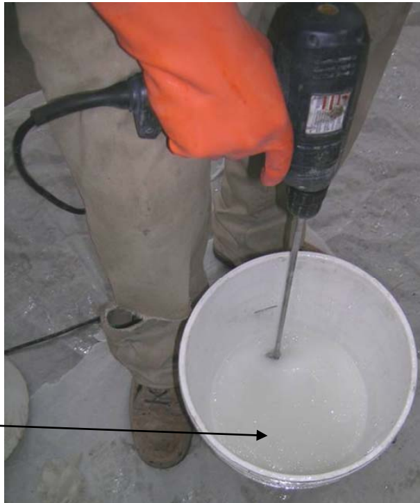
Figure 4.12 Mixing epoxy
