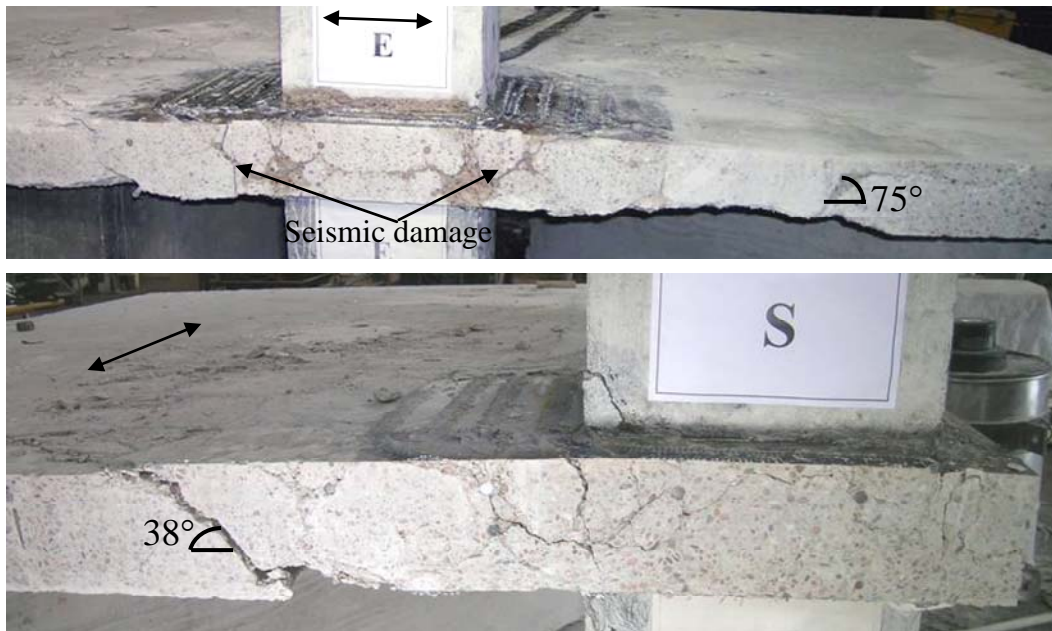
Figure 4.35 Failure surface of LRstG0.5
