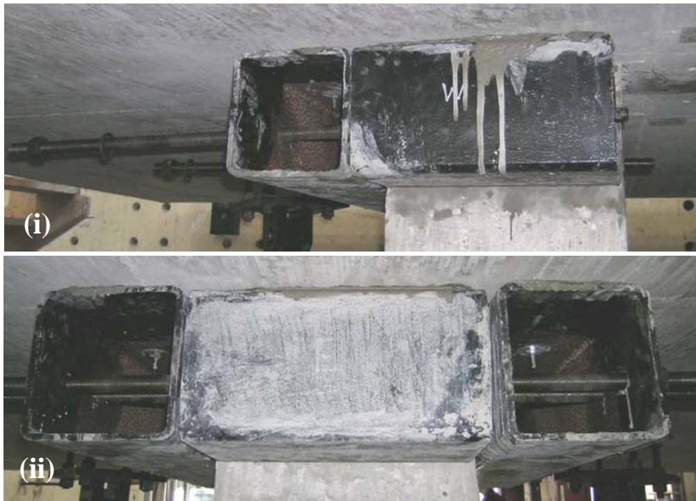
Figure 4.9 Installation of the longer steel tubes
