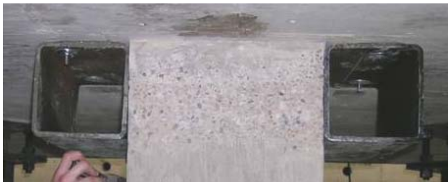
Figure 4.8 After installation of the shorter steel tubes
