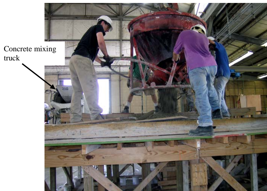
Figure 3.12 Concrete placement: slab and lower column
