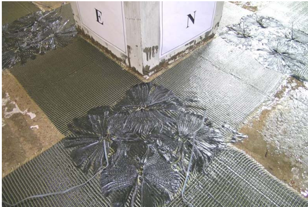
Figure 4.41 After installation of CFRP sheets and CFRP anchors
