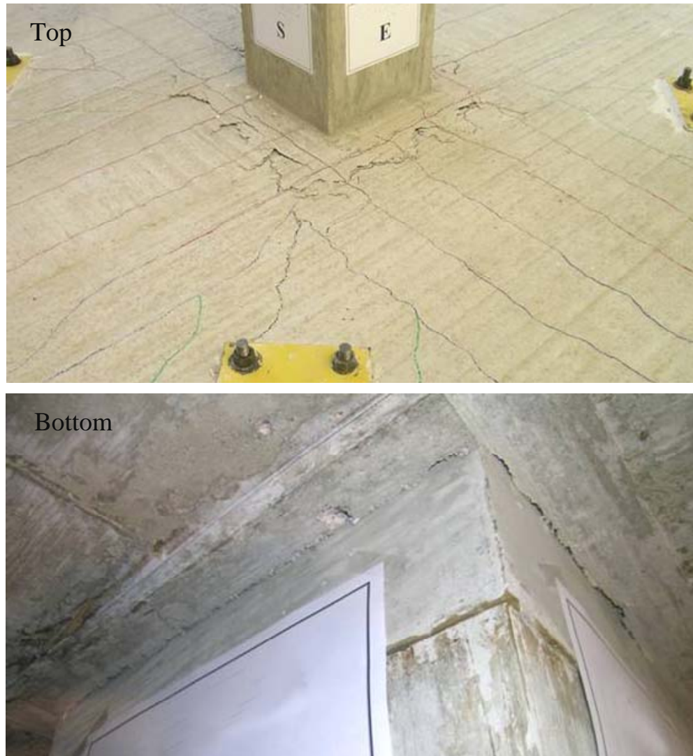
Figure 4.1 Failure surface of specimen G0.5
