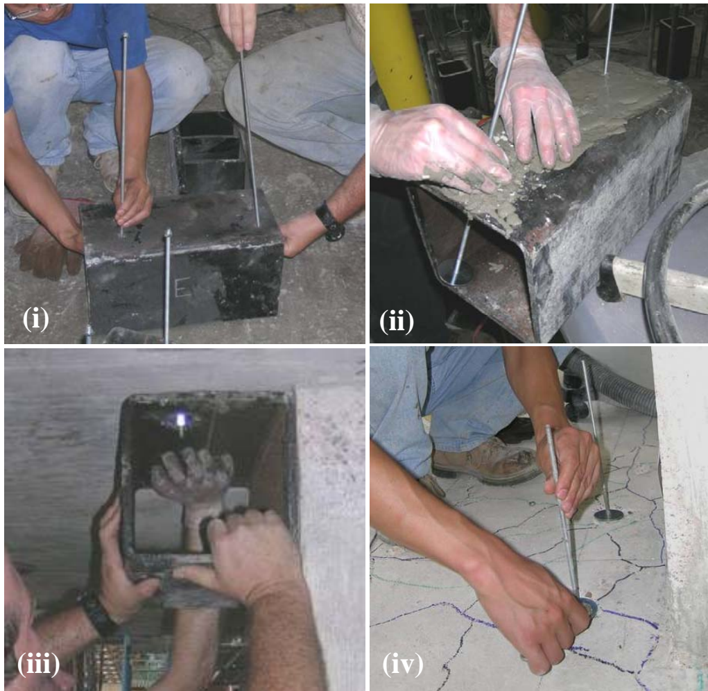
Figure 4.7 Installation of the shorter steel tubes
