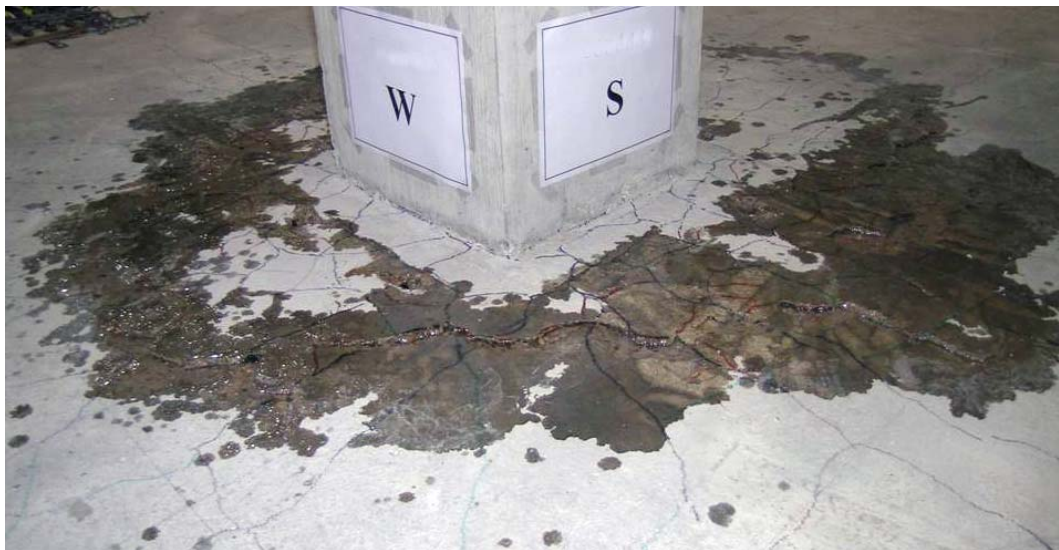
Figure 4.52 After epoxy pouring in RcL1.0
