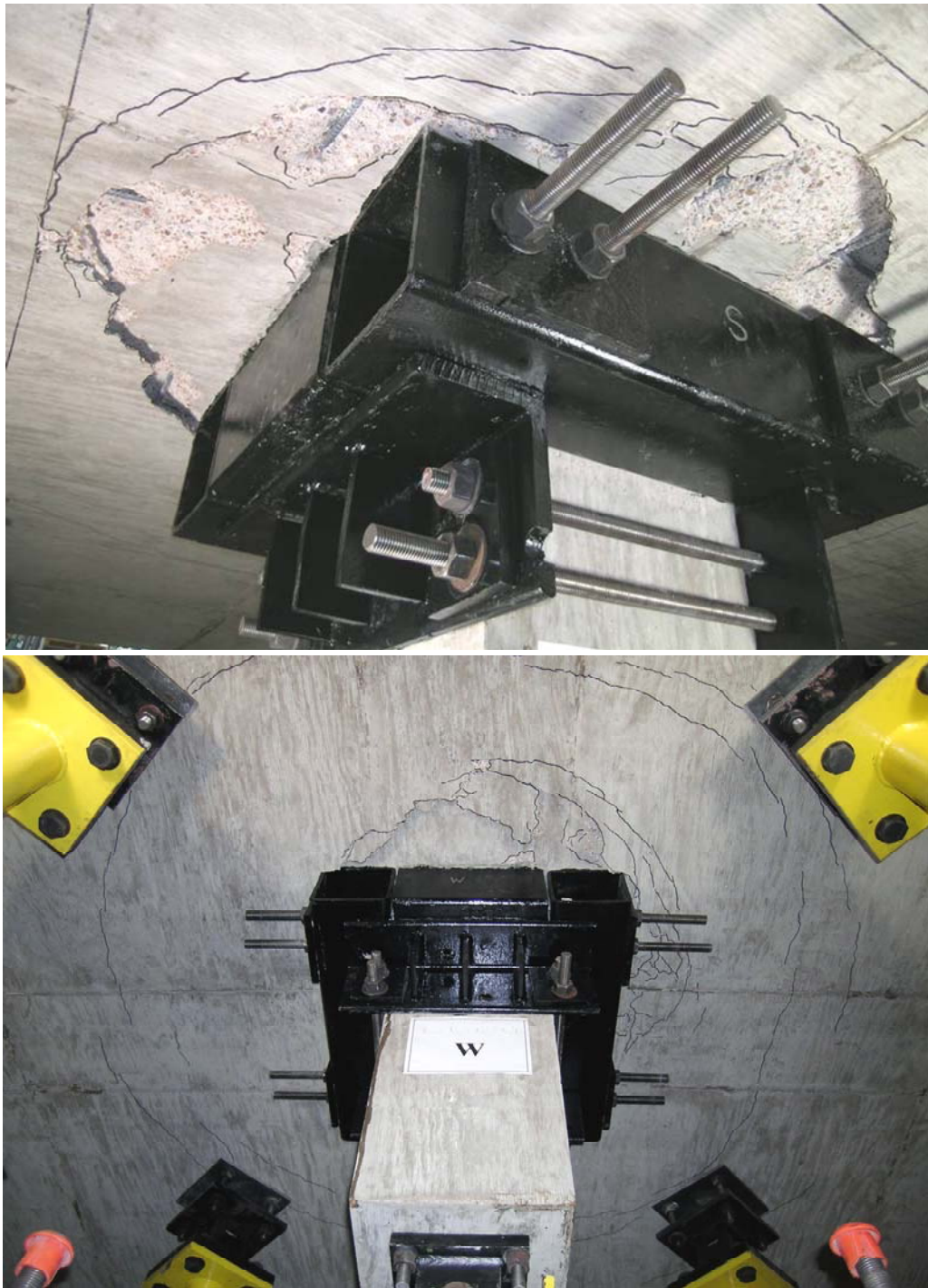
Figure 4.16 Bottom view of the failure surface of RcG0.5
